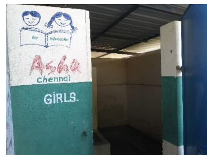
School toilets and washbasins funded by Hyundai Glovis
